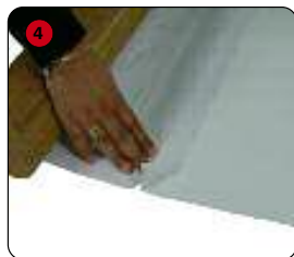
4 Align and adhere the adhesive leader to the bottom of graphic. (attach to back of graphic)
