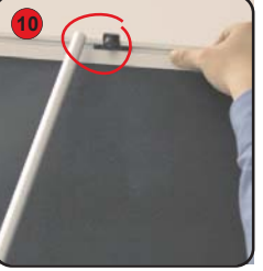
Finally, bend the bungee pole forward slightly and fit to the top rail.
