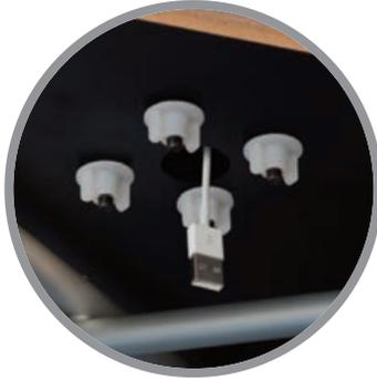
Feed USB end of charge/sync cable through middle of enclosure, below pin, so it protrudes from underside of counter/table top.
